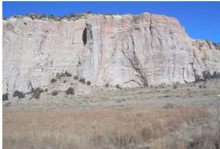
Figure S-3: Photo of cliff face near road (see Figure S-4) in El Malpais National Monument ( http://www.nps.gov/elma/index.htm ) in New Mexico.
